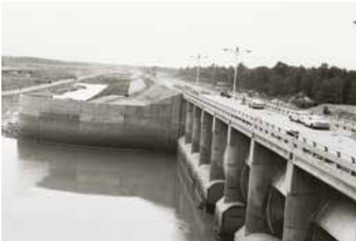
Spillway at the newly impounded Ross Barnett Reservoir in 1965.
