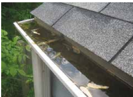
One of the best ways to prevent mosquitoes from breeding on your property is to remove standing water, such as in clogged gutters.
