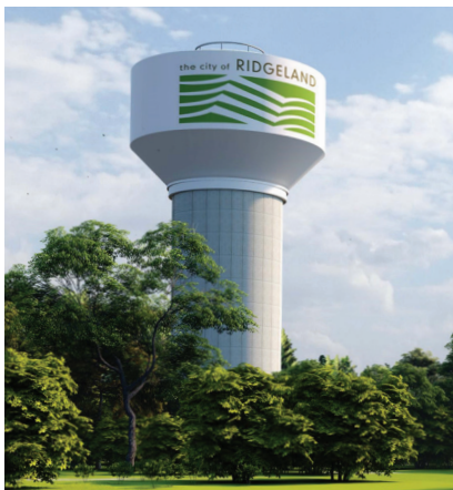
IN THIS PHOTO: A rendering of the soon-to-be-completed Water Tank
